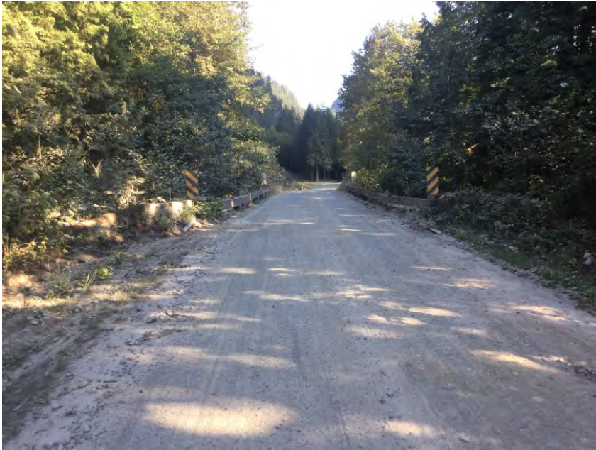
Right Approach Facing Bridge
