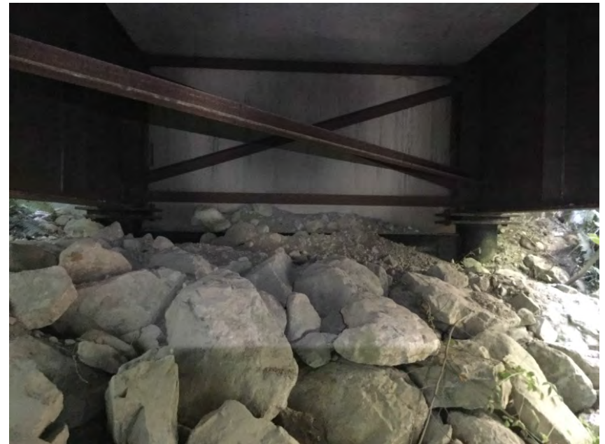
Right Bank Abutment
