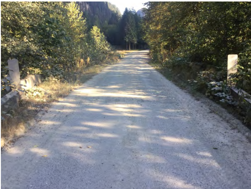
Left Approach Facing Away From Bridge
