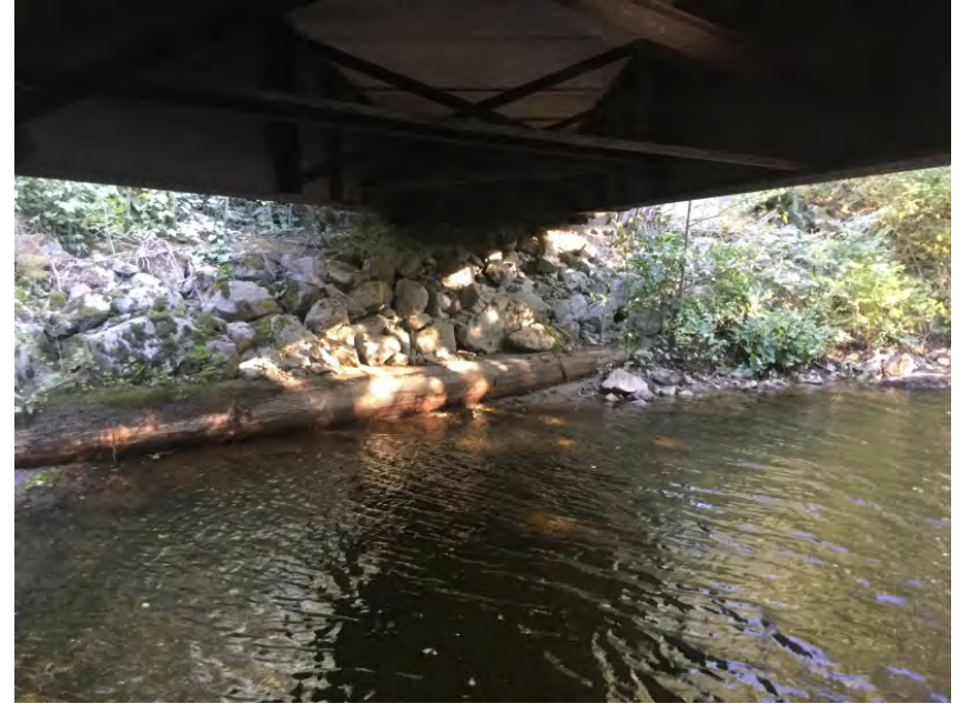
Left Bank Abutment
