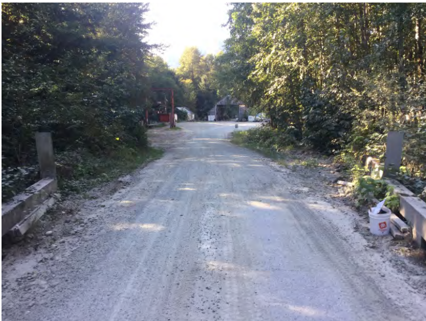
Right Approach Facing Away From Bridge
