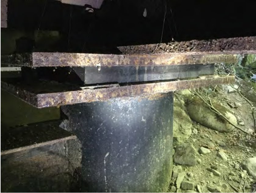
Typical Right Abutment Bearing
