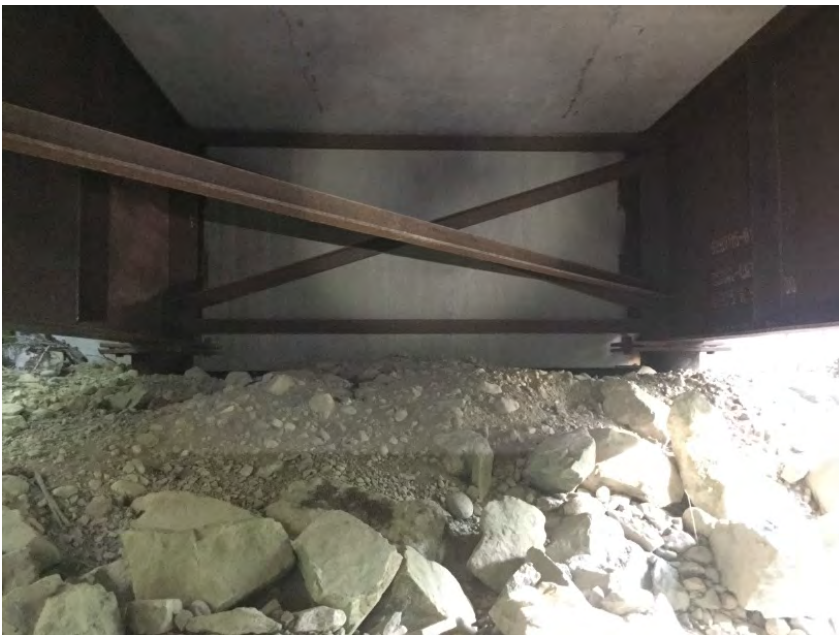
Left Bank Abutment
