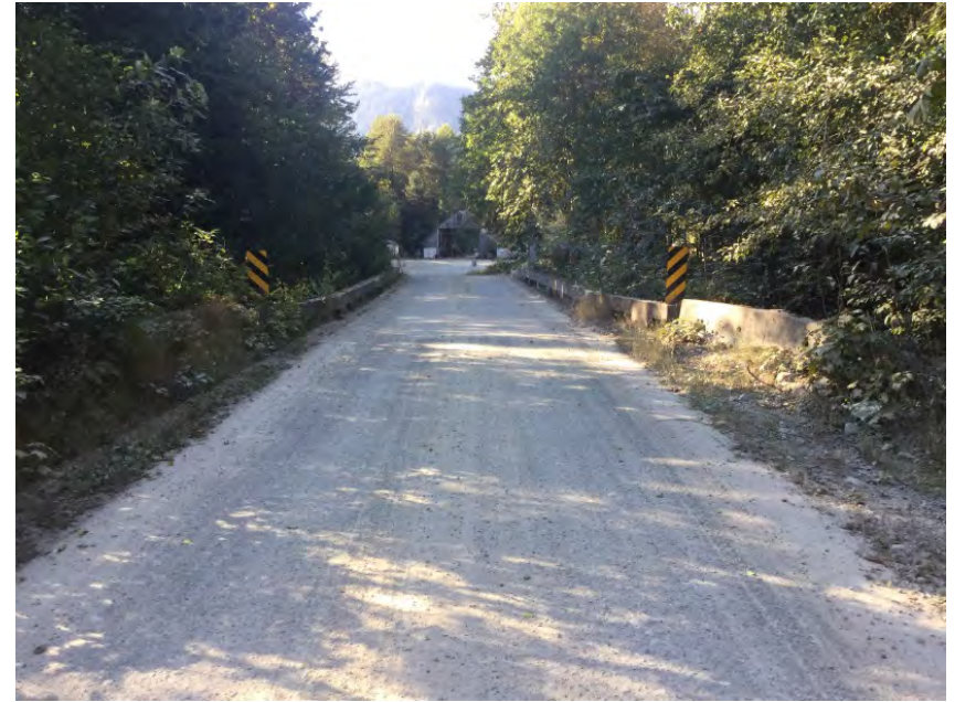
Left Approach Facing Bridge
