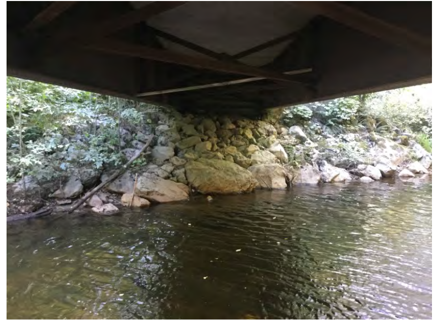
Right Bank Abutment
